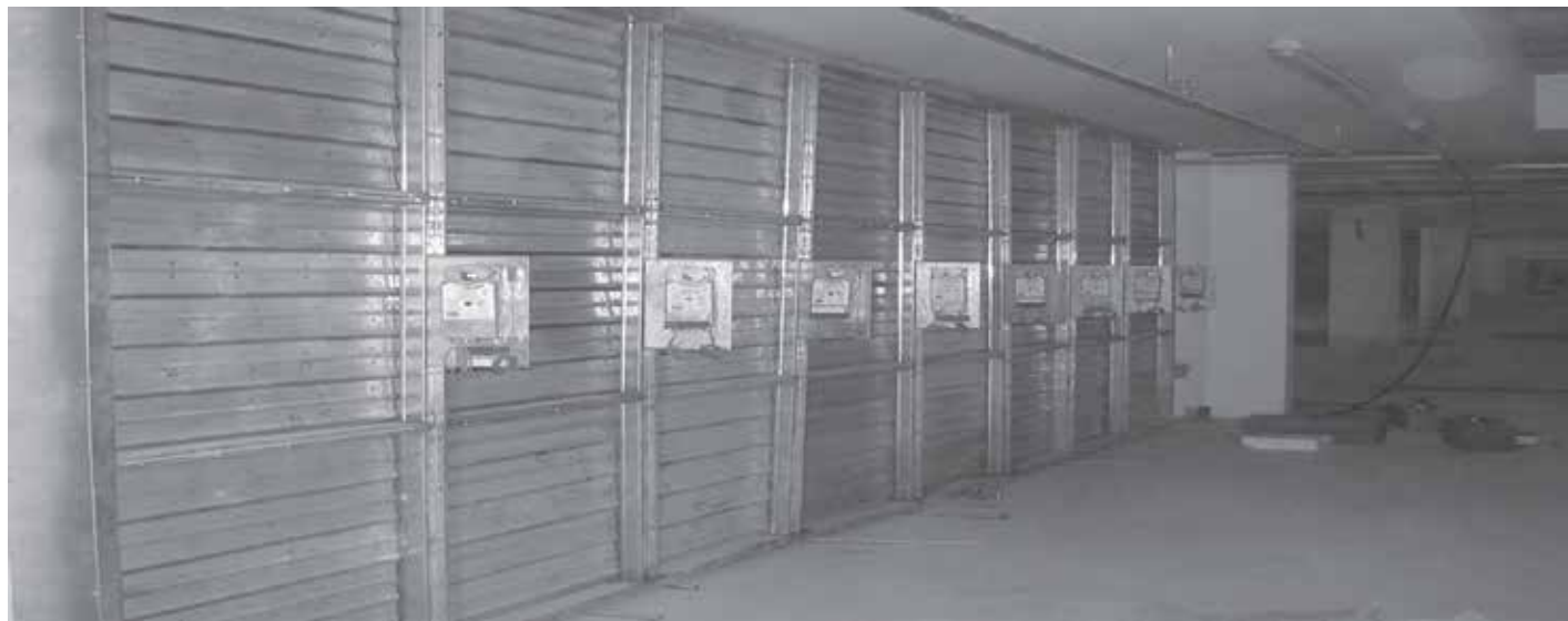
Multiple Damper Installation on site. Picture : Courtesy - Jebel Ali Down Town Site - Dubai - U.A.E
